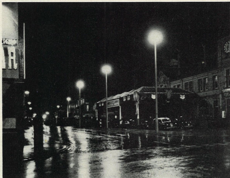
Fig. 3. Solacolor high pressure sodium lamps by Osram-G.E.C. have been operating experimentally outside Blackpool North Station since last July. The installation, consisting of six G.E.C. post-top type lanterns, each housing three 400W lamps, was planned by Blackpool's Engineer, Mr. H. Carpenter, F.I.E.S., M.I.E.E.
