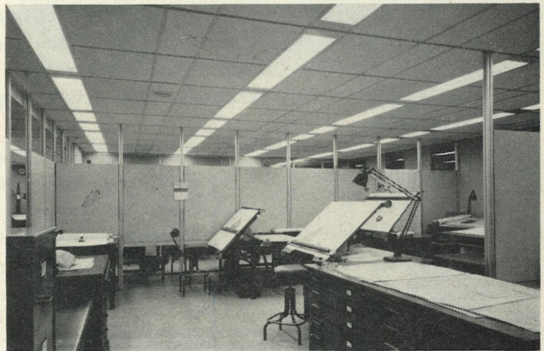
Office lighting on premises of Messrs. Tileman Estates Ltd
