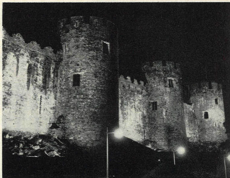
Fig. 4. Trial floodlighting installation at Conway Castle. Four trough floodlights for close offset and two narrow beam projectors for longer throws are employed.
